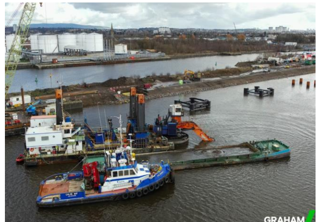
Image showing the dredging at Layby Berth
