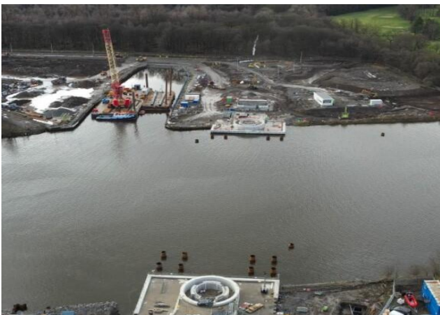
Image showing North and South Pivot Piers
