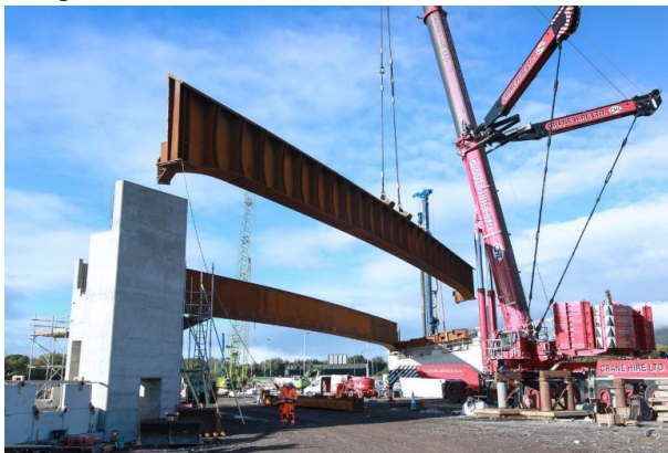
Image 1 Installation of Bridge Girders using 800t Mobile Crane
