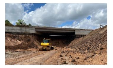
The excavated material will be hauled and used to form the embankments for the new Adlington bridge, with large quantities also being used to complete the remaining earth bunds along the east side of the project. The completed bunds will help screen the new road and provide mitigation against traffic noise.
