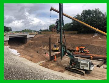
The works included the installation of 186 sheet piles to a depth of up to 10m, using a piling rig and hydraulic vibro-hammer machine. The piling machine transfers vertical vibrations to the sheet pile via a hydraulic clamp, loosing the soil and aiding the installation of piles. The team took the decision to pre-auger and excavate 6m into the ground ahead of the sheet pile installation, in order to minimise the vibration levels on our neighbours.
