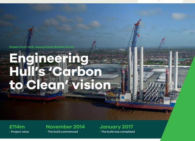
Featuring the maiden project of the world's largest dredger (Manu Pekka), one million tonnes of imported Norwegian Stone and one million cubic metres of sand, this major £114m redevelopment of Alexandra Dock has revolutionised the Green Port Hull's functionality. Part of a Joint Venture with Lagan Construction, our team creatively designed, and constructed, the Port to accommodate three offshore wind installation vessels on behalf of Associated British Ports' (ABP) end user Siemens.
